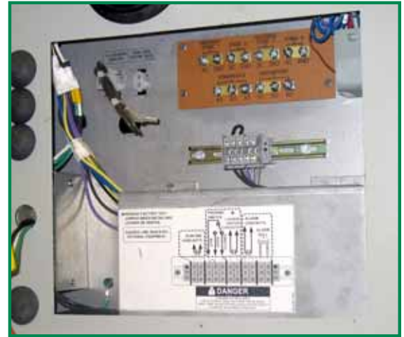
All BMS connections are on the front portion of the unit and have been designed for easier access and connection.
