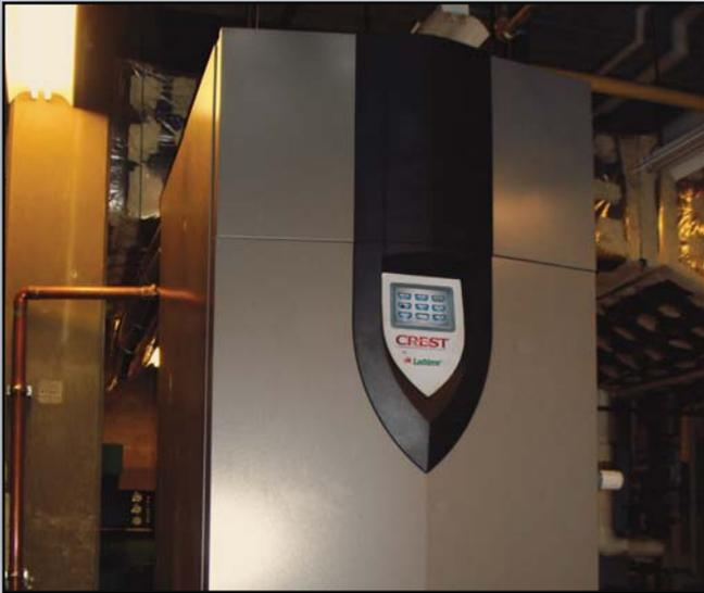
reset functionality, one of the many features offered with its exclusive SMART TOUCH™ operating control. Since outdoor reset adjusts the heating system water temperature based on the outdoor air temperature, it allows for decreased fuel consumption and increased consistent comfort.
