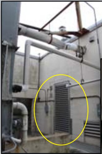
*Air louver fitted to fill the small access hole created to install the boilers.*
