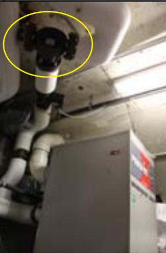
*Lochinvar LTV Valve protects the non-condensing Power-Fin from low return water temperatures. This increases efficiency of the system while protecting the boiler*
