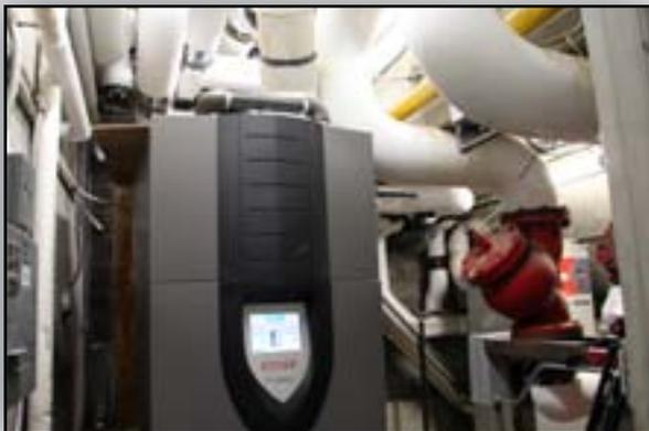
Despite the complexity of getting the boilers into the mechanical room, the CREST Boiler's SMART TOUCH operating control simplified the rest of the installation. Utilizing CREST's built-in cascading sequencer, the two boilers are operating in a cascade sequence as a front-end loading system. The CREST carries the load approximately 80 percent of the time, and the Power-Fin is brought on during the coldest days to help meet the largest heating demands.
