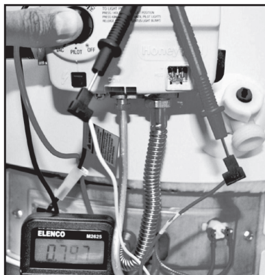
USE A MULTIMETER TO CHECK THE OUTPUT OF THE THERMOPILE (MEASURED IN MILLIVOLTS). SHOWN ABOVE - MULTIMETER PROBES ARE INSERTED INTO THE THERMOPILE PLUGS. THESE PLUGS WERE REMOVED FROM THE RECEPTACLE AT THE BOTTOM, RIGHT-HAND CORNER OF THE GAS CONTROL VALVE/ THERMOSTAT.
