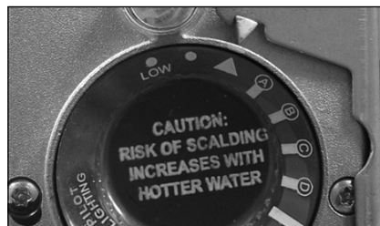
Figure 37 - Adjust the gas control knob to "▲".
