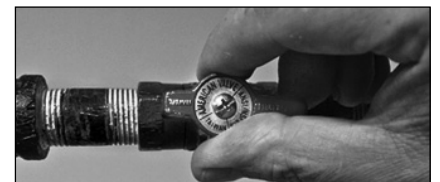
Figure 50 - Gas valve in "on" position.
