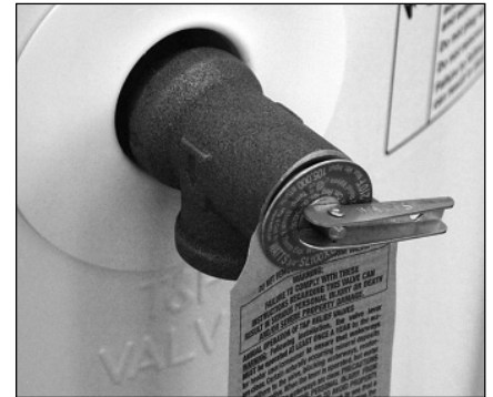
Figure 25 - Temperature and Pressure Relief Valve
