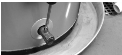
Figure 40 - Draining the water heater.
