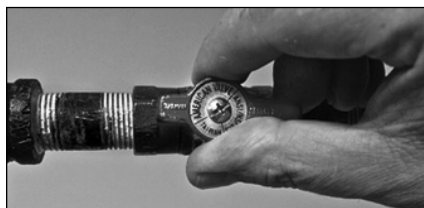
Figure 32 - Gas valve in "on" position
