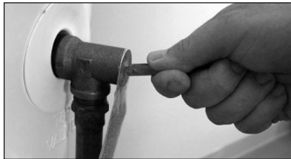
Figure 43 - T&P Relief Valve.
