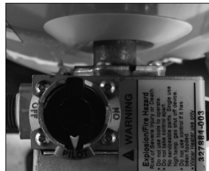
Figure 34 - Gas control/valve top view.
